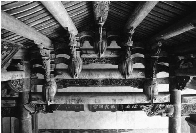
Figure 2.14. Dié-dǒu wood framing system. (After Lin, 1990: 64)
