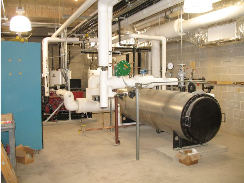
BioDiesel Engine Generator with Heat Recovery Equipment, MMCH C9
