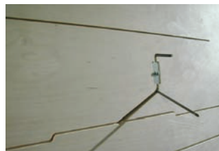
figure 8. back lighting at panel
