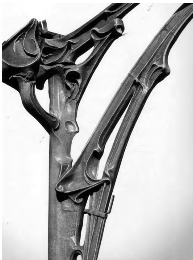
Figure 30 Ironwork connection detail between column and Métro sign
