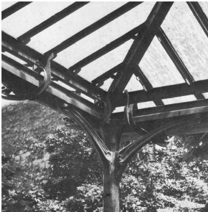
Figure 32 Column-roof detail inside Porte Dauphine station
