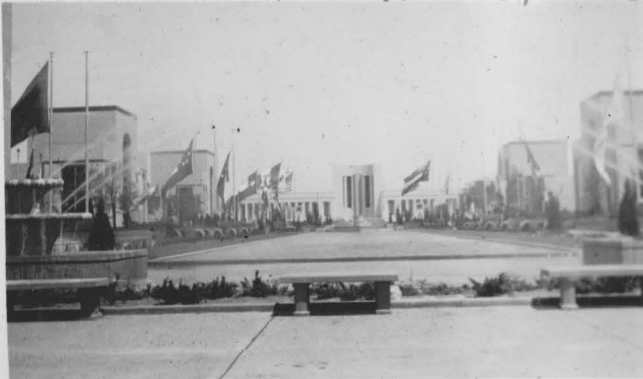
TEXAS CENTENNIAL - DALLAS, TEXAS
