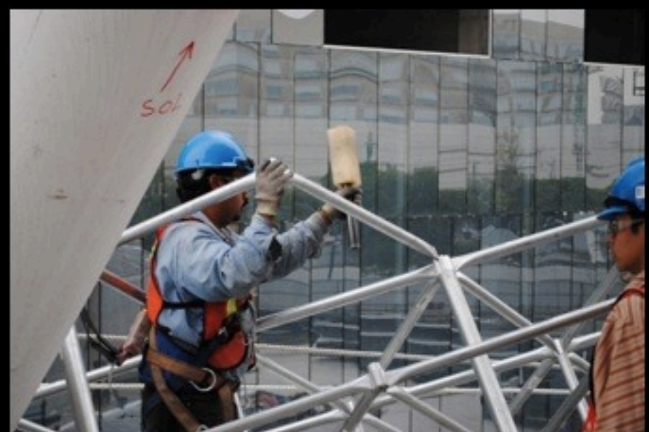
Secondary Structure Assembly
