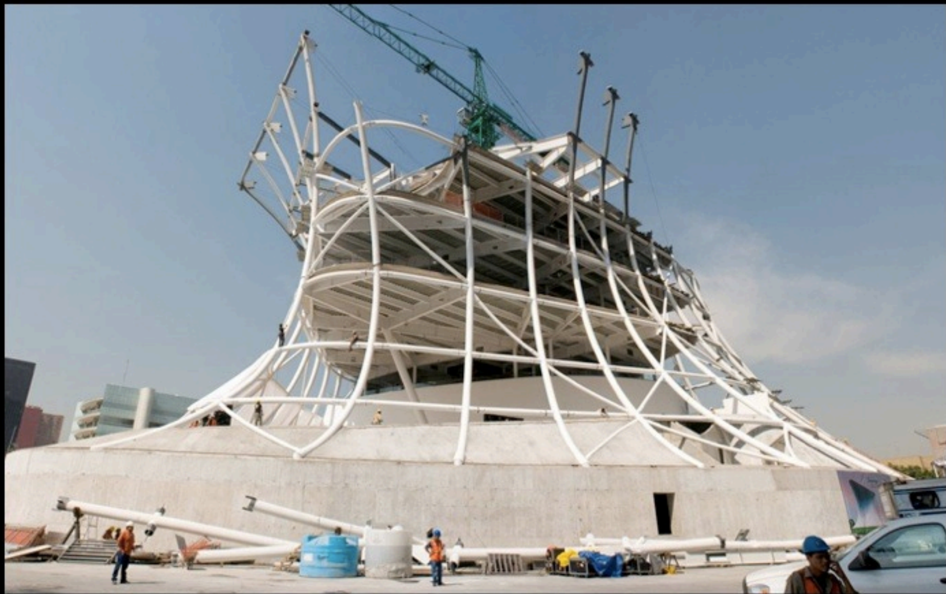
Primary Structural Frame: 52cm dia Steel Pipe
