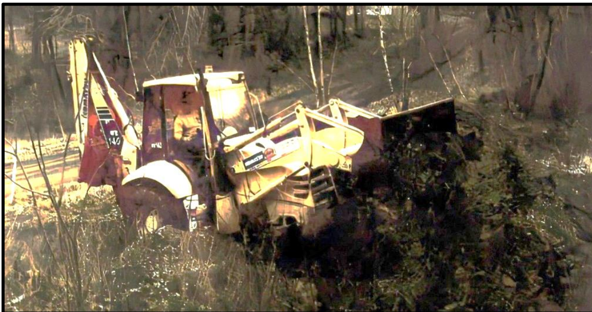
Figure 50. Contractor blocking coal road to discourage dumping. Standard Speaker Jan. 17, 2007
