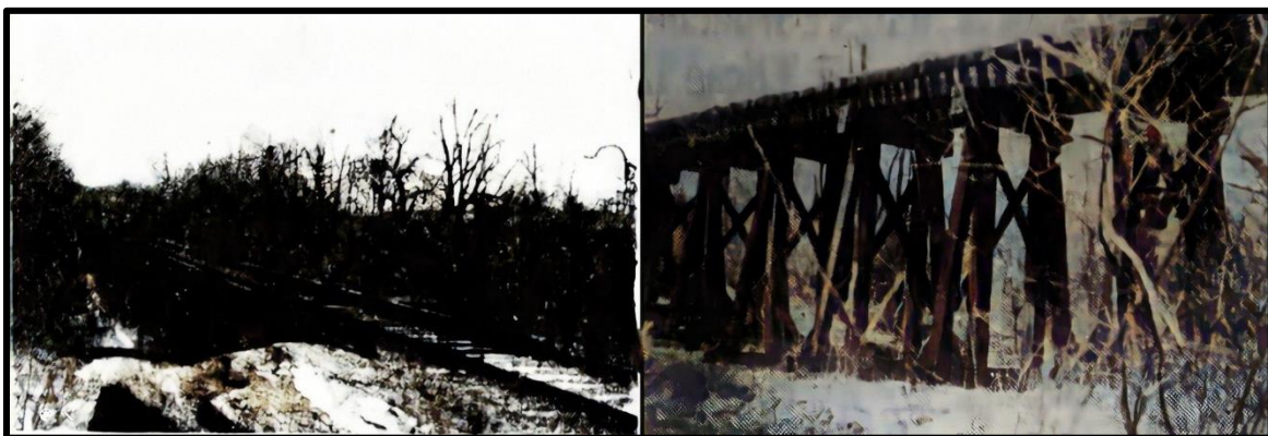
Figure 40. Upper Lehigh CRRNJ rails and trestle 1959. (Hazleton) Standard Speaker
