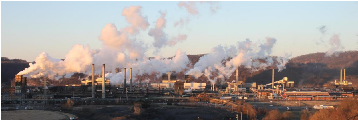
Figure 1.8: A photo showing the operation of the U.S. Steel's Clairton Coke Works [59]. After being released from the plant, SO 2 travels in the form of a plume that widens with distance from the plant. SO 2 exits the stacks with a much higher temperature than that of the ambient air.
