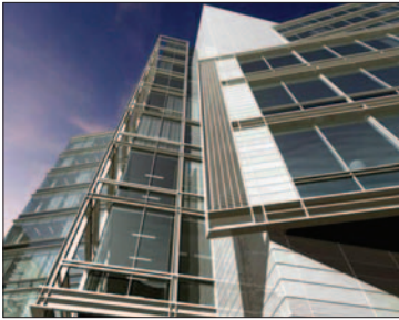
Image courtesy of Burt Hill Kosar Rittelmann Effectively communication design intent before construction.
