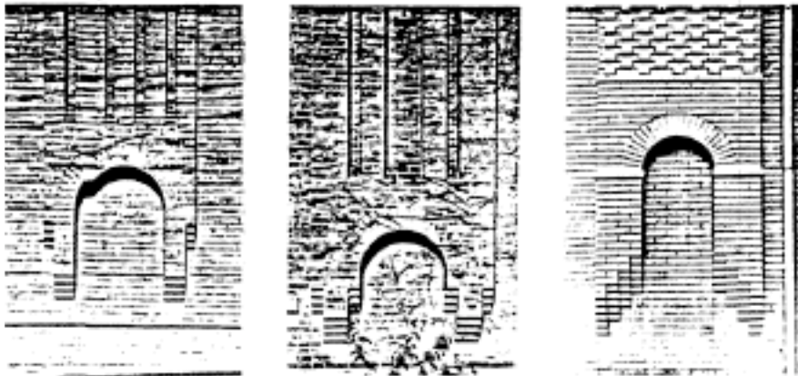
Figure 21. Bottom ends of chimney breasts.
