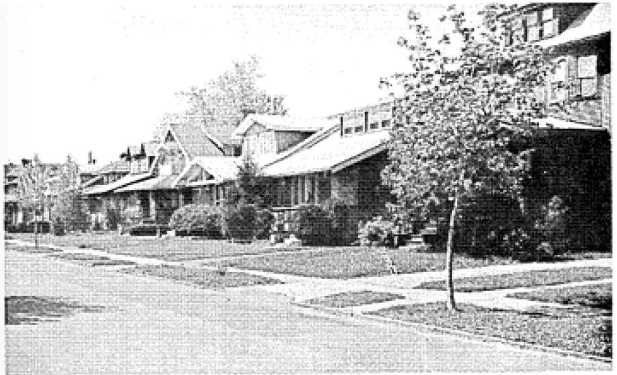
Street 1 and five bungalows
