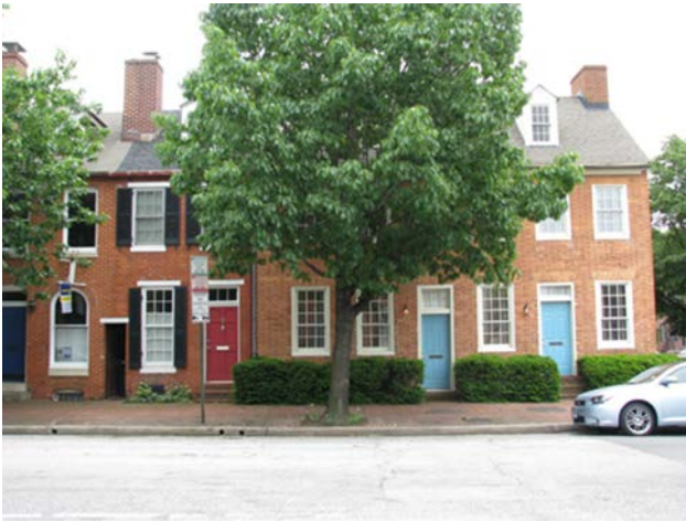
(a) 1-11 East Montgomery Street (1 is on the right)
