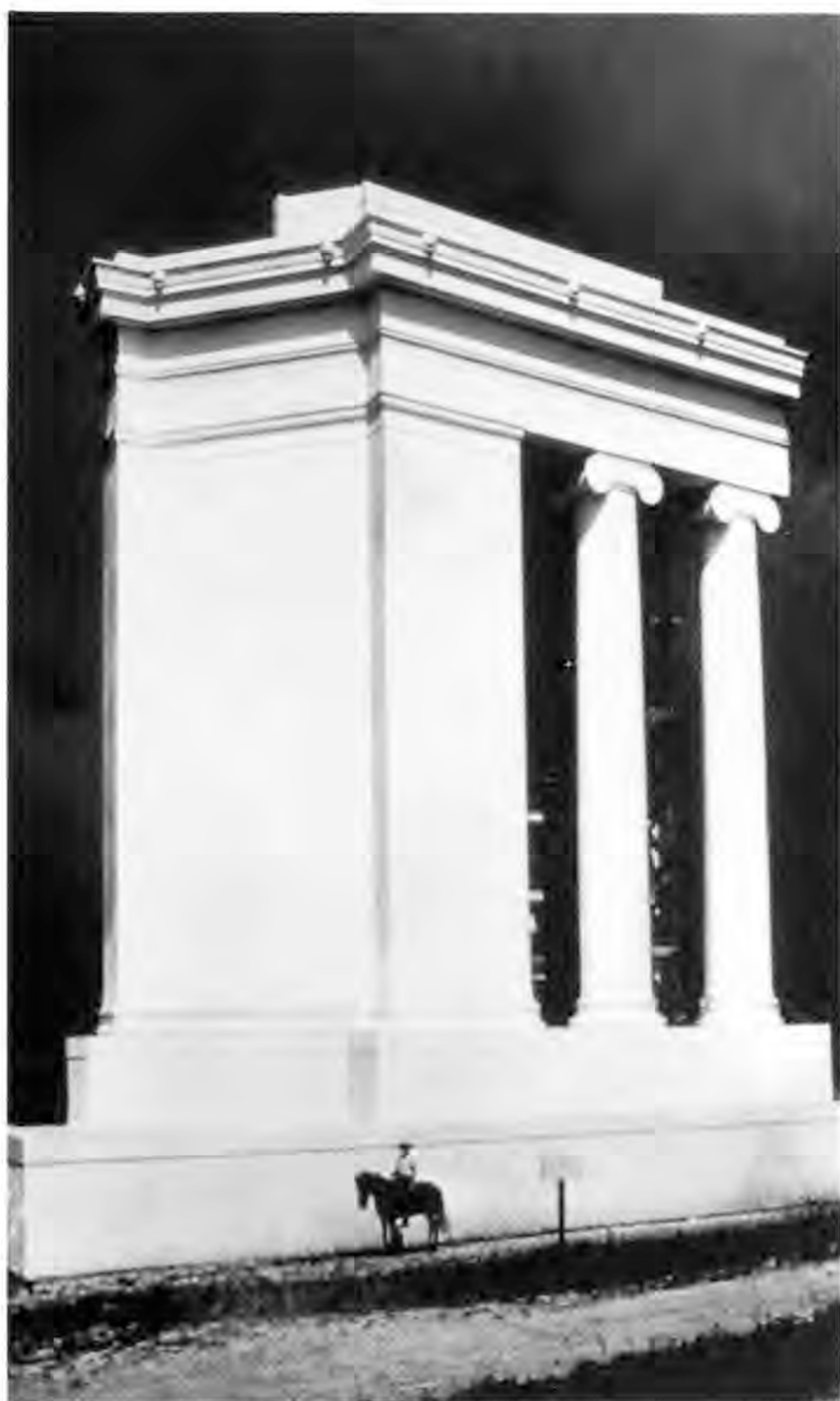
Mellon Institute's focus on experimentation was applied in the design of its own new building. In 1931, a full-scale model of a corner pier and two columns were erected in Fox Chapel, and studied for 19 months.
