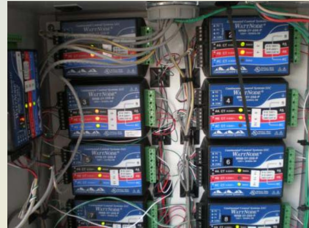
WattsNode connecting with CTs
