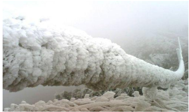
Figure 1 icing cable in storms, Guangxi, China 2008-02-02 16:26:29
