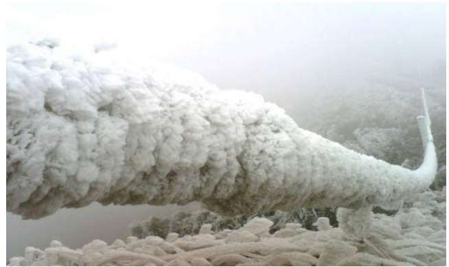
Figure 1 icing cable in storms, Guangxi, China 2008-02-02 16:26:29
