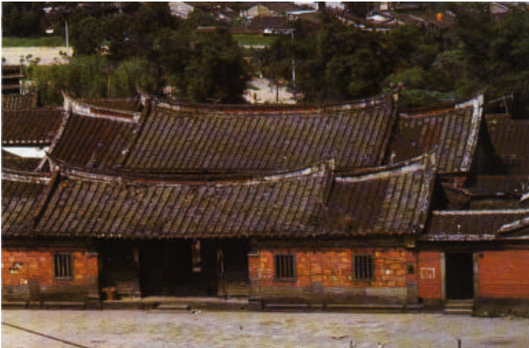
Figure 26. The Lín Ān-tài residence. (After Li, 1980: 126)
