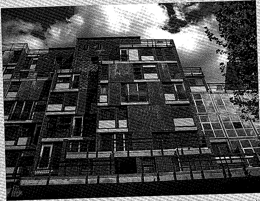
Figure 4.3 La Maison Médicale (La Mémé) in Woluwe-Saint-Lambert, Brussels: Lucien Kroll designed the exterior as a framework such that students could create and change their own façade by choosing among its various finishes, sizes, and removable panels. Image (and text) courtesy of Kush Patel, PhD student, University of Michigan Taubman College of Architecture and Urban Planning.
