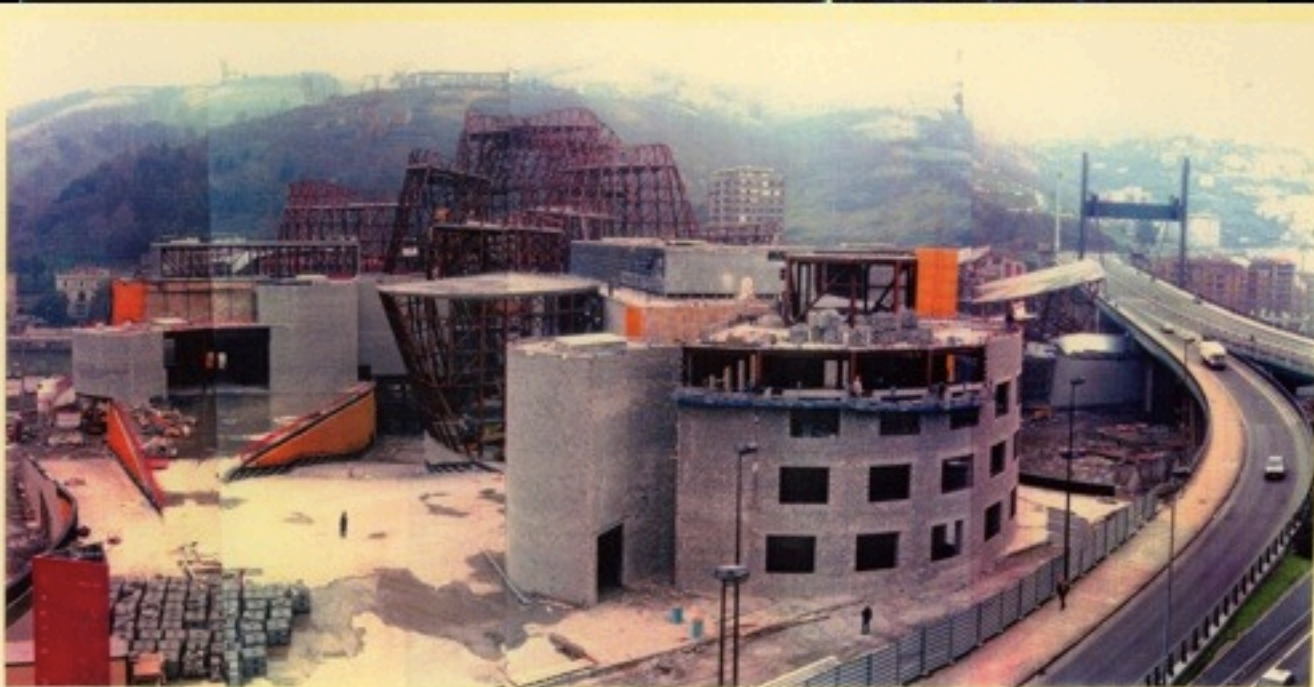
Construction: Steel Frame & Masonry Back-Up System
