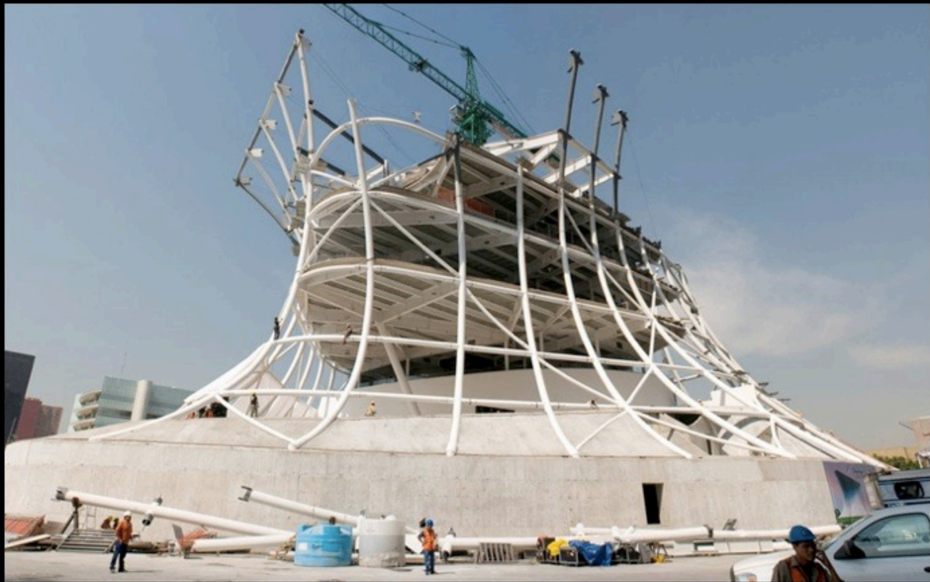
Primary Structural Frame: 52cm dia Steel Pipe
