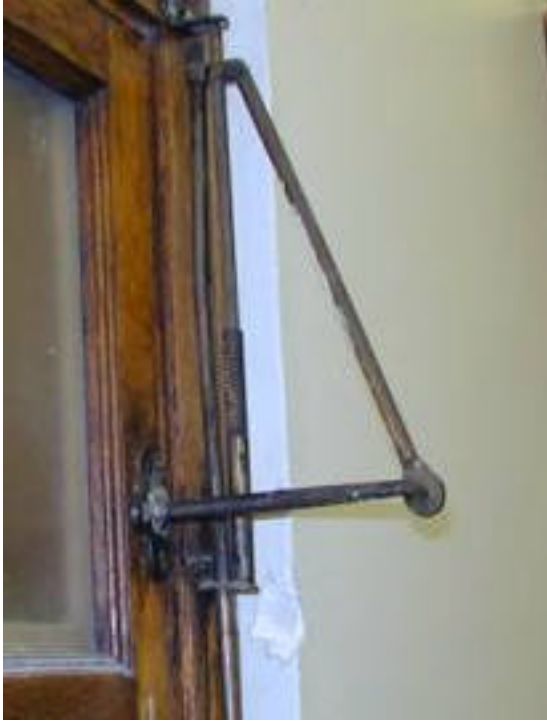
Fig. 1 Mechanism in the closed position.
