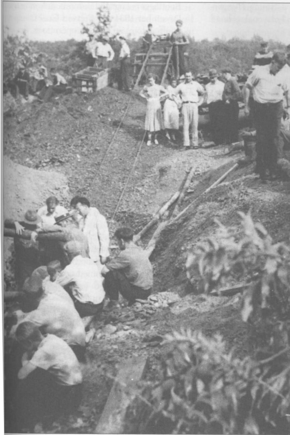
Figure 3.7: Photograph of a 1936 bootlegging accident at a small mining town called Wiggans Patch. Note the large number of civilian rescuers and onlookers and the very basic technology being used to extract the miners. Since bootlegging was illegal, area residents were left to their own devices to deal with problems when they occurred. Image from Dublin and Lich, The Face of Decline , p.77.
